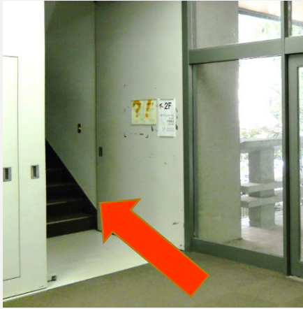
Stairs at the very back of the first floor.
